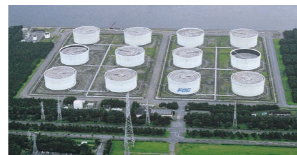
Crude oil tanks at the Nakasode Crude Storage Base
