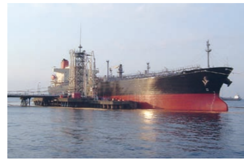
Dedicated landing pier Capable of handling tanker up to 120,000 DWT
