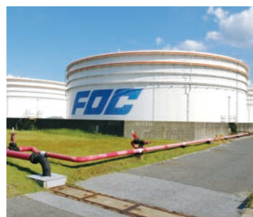
Crude oil tanks at the Sodegaura Refinery
