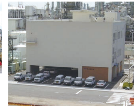
Integrated control room
