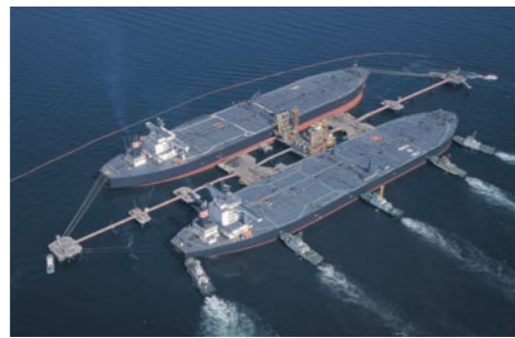
Keiyo Sea Berth Located 7 km offshore from the Sodegaura Refinery, the sea berth can accommodate two 300,000 DWT tankers concurrently. The sea berth is connected to the Refinery by an undersea pipeline.
