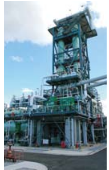
Low-exergy generation system
