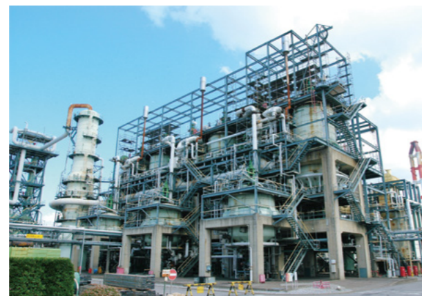
Vacuum residue thermal cracking unit (Eureka Thermal Cracking Unit)
