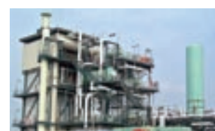
New hydrogen production facility
