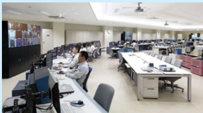
Integrated control room
