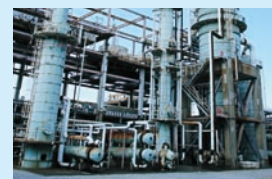
Crude Distillation Unit (CDU)
